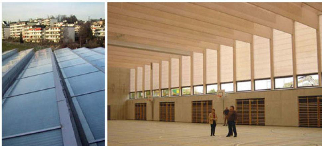
Roof Construction Application Examples of Granular Aerogel Filled Glass Fibre Composite Panels Produced by Cabot Corporation (Koebel et al., 2012)
