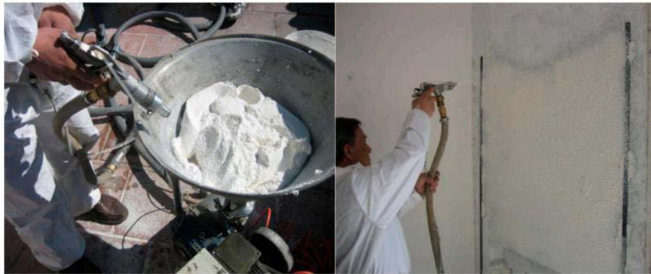
Application of Silica Aerogel Reinforced Plasters (Buratti et al. 2014)
