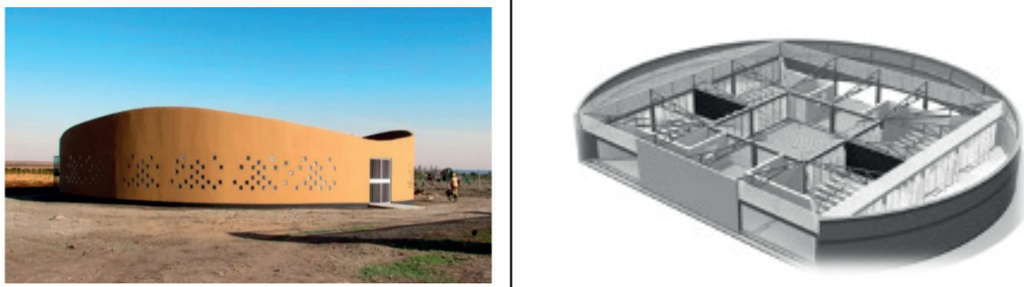
Figure 6. The Uaso Nyiro primary school's water collection system
